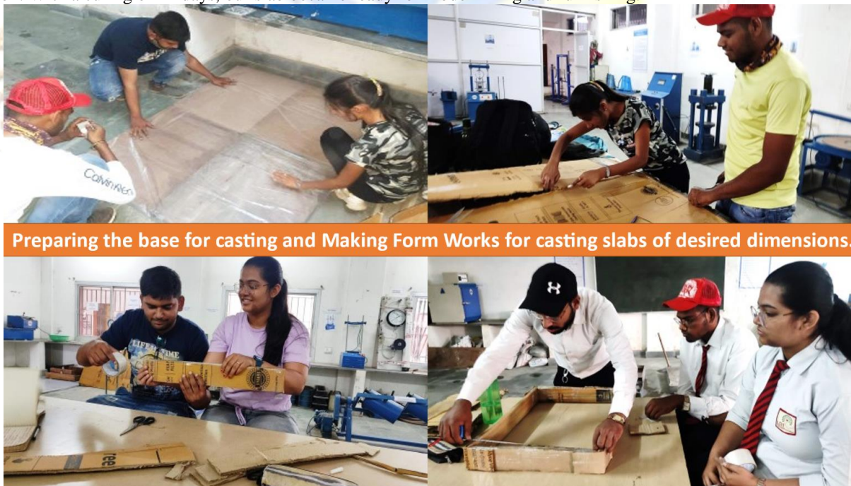
Fig 13 Preparing base for slab casting & Making strips for Form Works
