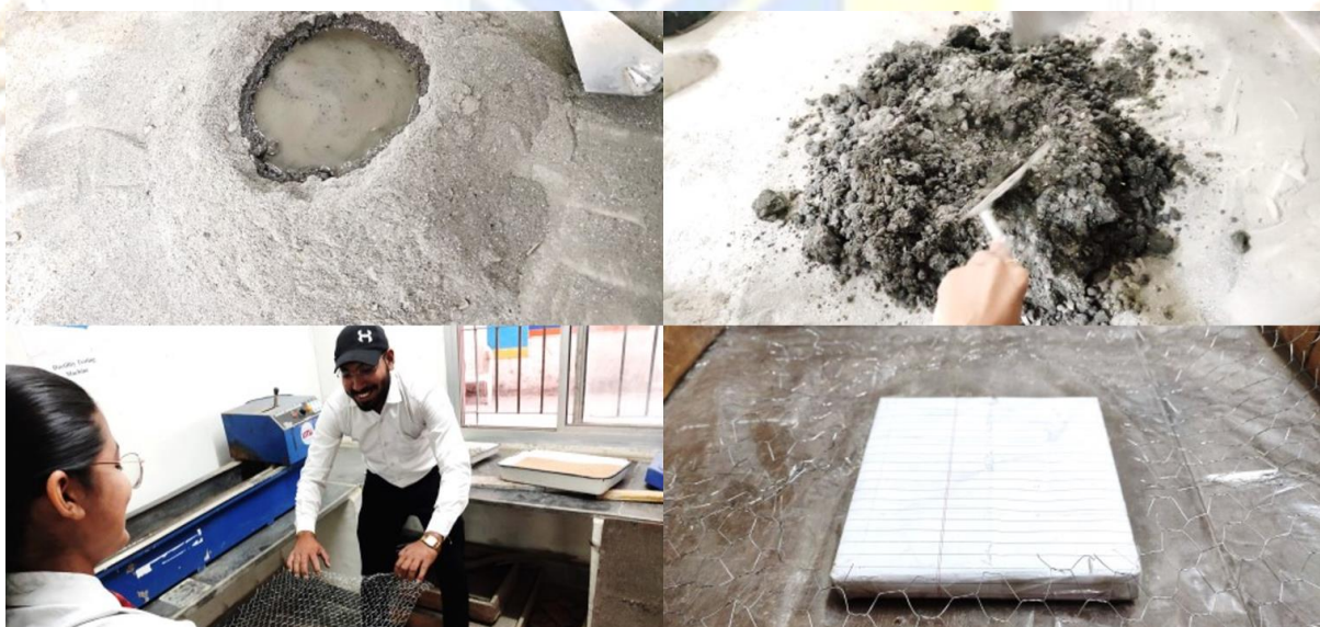
Fig 16 Preparing Concrete mix, placing wire mesh and open space blocks.
