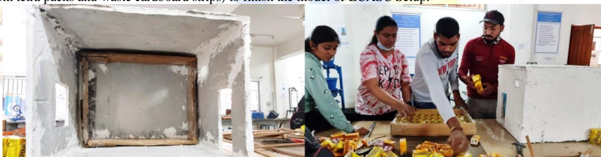
Making Stackable Structure Using the Form works themselves and stacking filled Tetra Packs.
