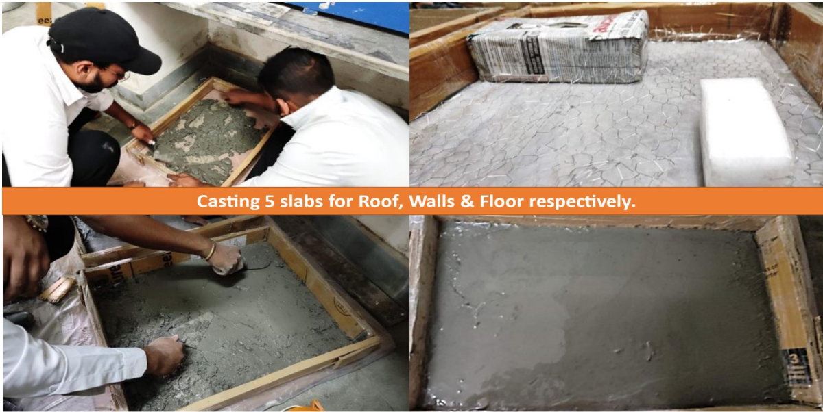
Fig 17 Slab Casting
