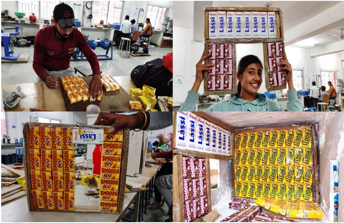
Fig 22 Making Stackable Structure with filled Tetra Packs
