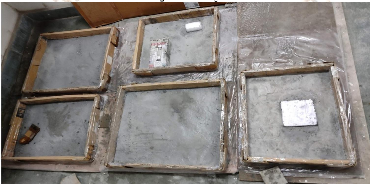
Fig 18 Casting slabs with proper compaction and surface finish
